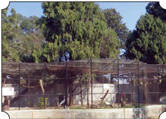
Newly constructed Aviary
