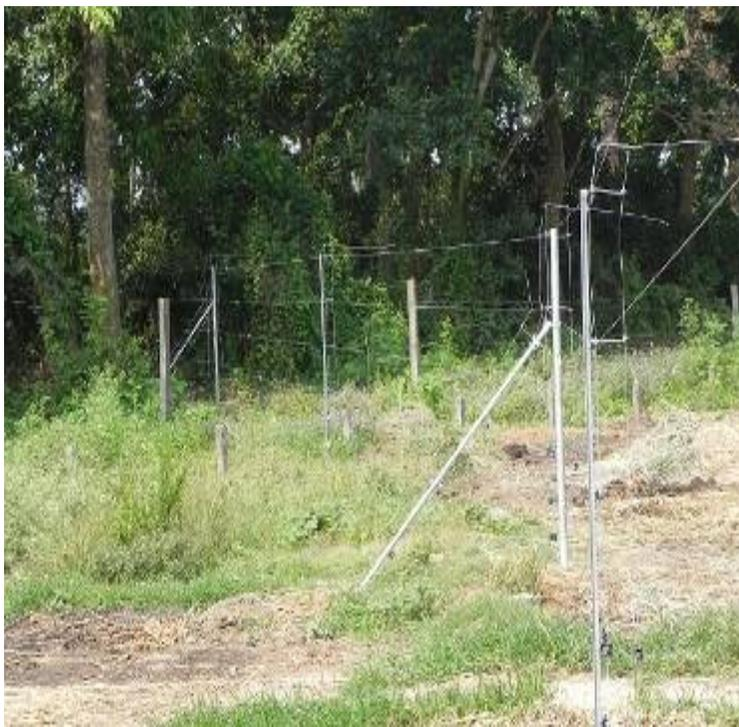
The corrals stand seven feet tall, constructed of rust-free steel posts and six strands of high tensile wire.
