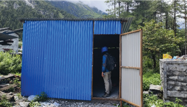
Photo: Waste collection recently constructed at Kalopani
